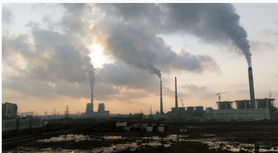
Jiangsu Nantong power station, 2016. Photo courtesy of Kristoferb .
